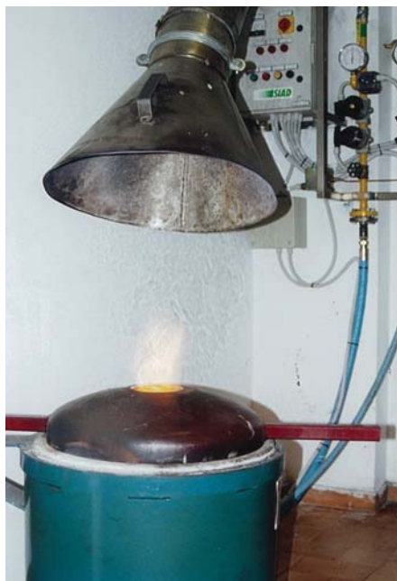
Crucible furnace with O 2 -CH 4 burner.
