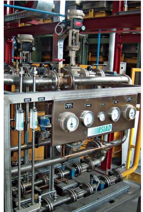
*Oxy-fuel unit for rotary melting furnace*
